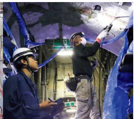
Concrete structure maintenance (STTG method)
