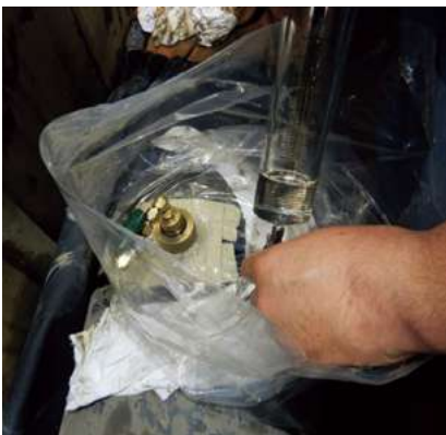
OF cable insulation oil sampling
