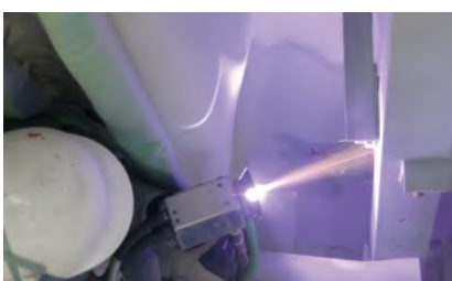
Antirust thermal spray method
