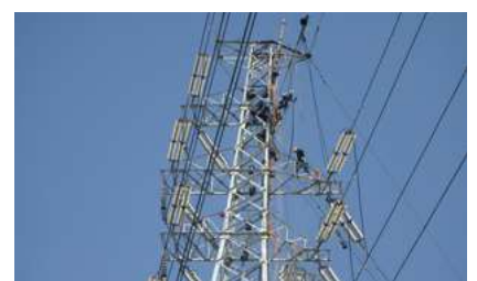
Replacement of deteriorated steel
