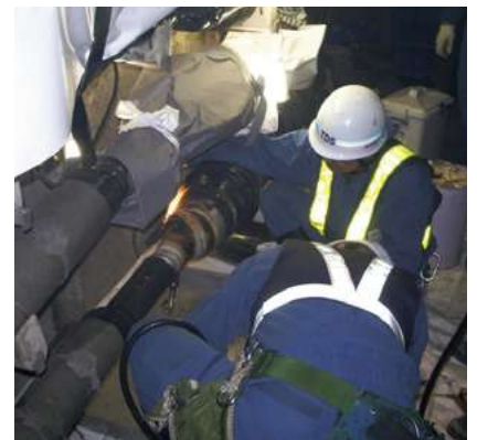
OF cable oil leak repair
