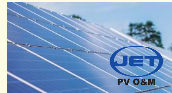
Registered as a Photovoltaic System Maintenance and Inspection Contractor under the JET certification system
