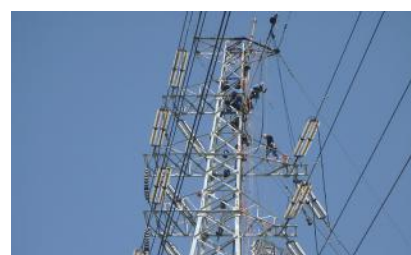
Replacement of deteriorated steel
