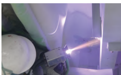
Antirust thermal spray method
