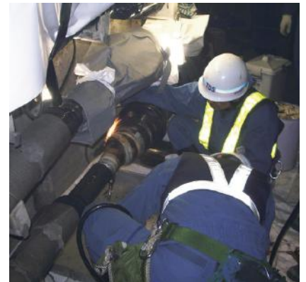
OF cable oil leak repair
