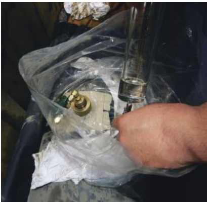
OF cable insulation oil sampling
